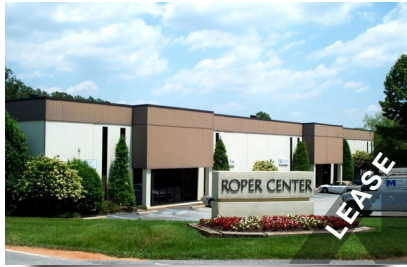
6021 Ponders Court | Greenville, SC 9,200 SF Earle Furman, SIOR & Jon Good, SIOR
