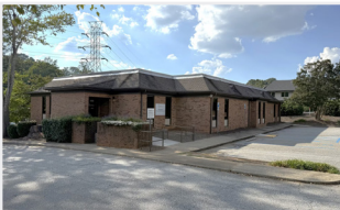
1350A Cleveland St Greenville, SC ±8,464 SF
